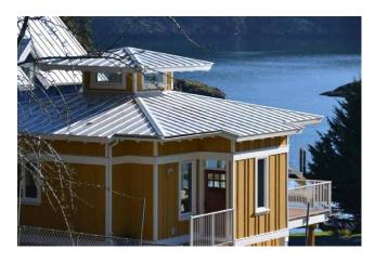
**Non-Porous Material** – Metal is a non-porous material and can withstand freeze and thaw cycles without damage, degradation, or deformation, making it ideal for snowy environments.
